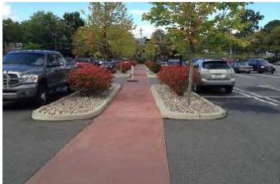
Figure 5.14.d.4.c.ii Parking lot pedestrian paths. Another example of a dedicated parking pedestrian path through a parking area
