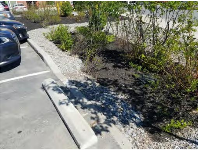
Figure 21. Stormwater retention. Use of creative stormwater retention designs can allow for landscaped areas to absorb rainwater locally and filter it without it having to be piped underground, where it can pollute the local waterways. This design has a lowered curb edge which allows the rainwater to flow down into the lowered planting bed where it can be absorbed by the ground and provides water for the plants. A hidden overflow pipe allows excess water to escape to prevent overflow.
