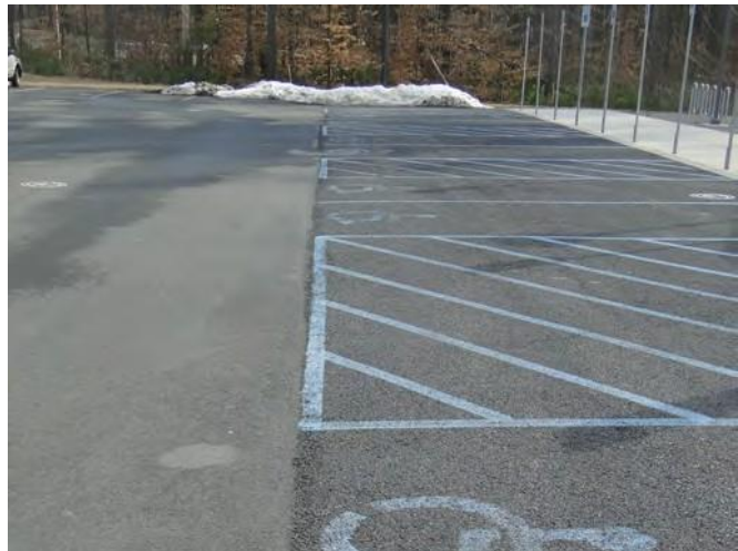
Figure 56. Porous pavement. Utilizing porous pavement helps to limit the amount of stormwater runoff from a large parking area.
