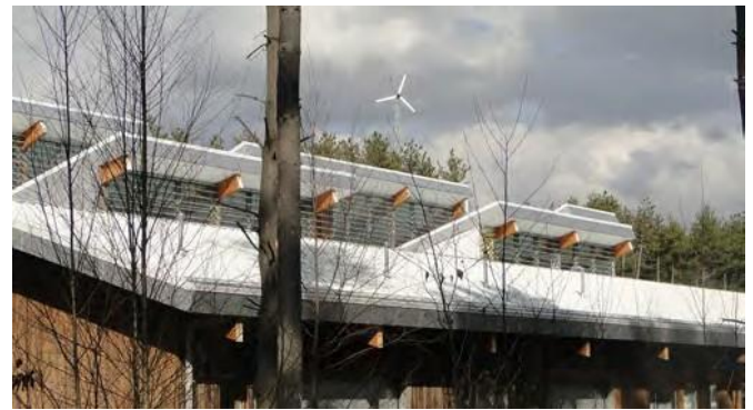
Figure 58. The rooflines of this building are broken up with the use of interesting clerestory windows which also help to bring natural light down into the center of the building.
