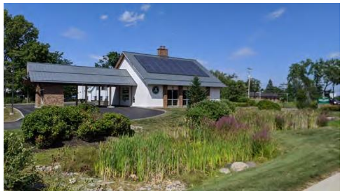
Figure 26. Stormwater retention pond at a commercial bank designed to look like a natural area.
