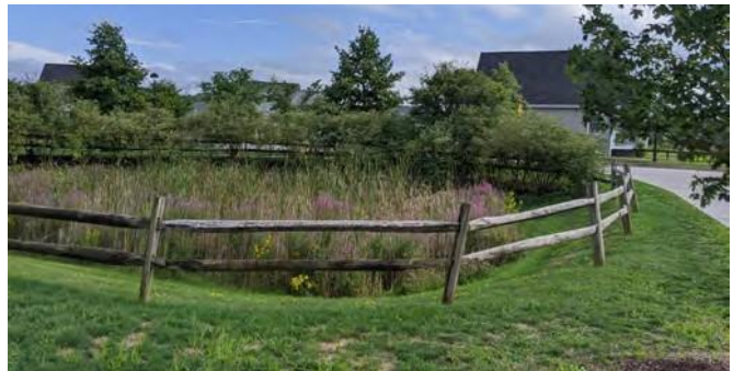
Figure 25. Stormwater retention pond in a housing development designed to look like a natural pond.
