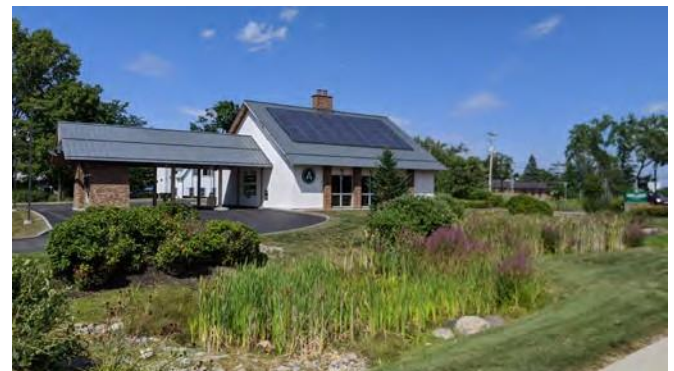
Figure 26. Stormwater retention pond at a commercial bank designed to look like a natural area.
