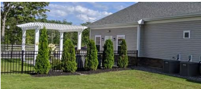
Figure 27. Screening of mechanical equipment.
