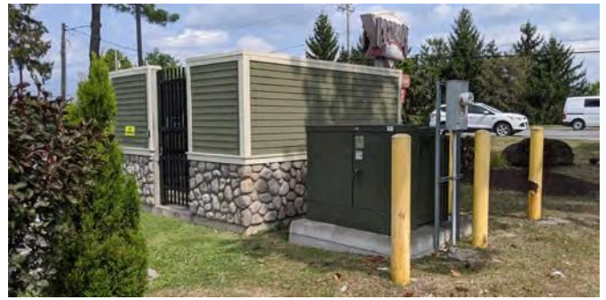
Figure 28. Screening of mechanical equipment.
