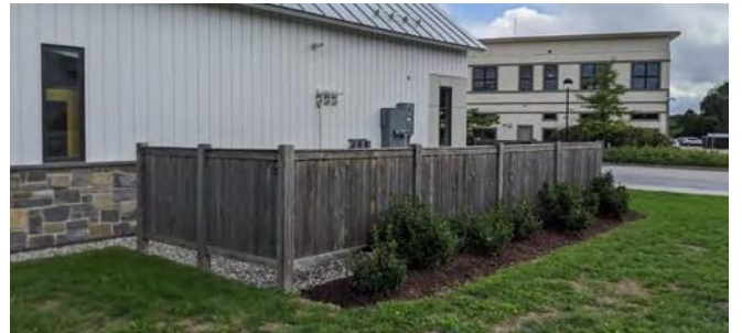
Figure 29. Screening of mechanical equipment.
