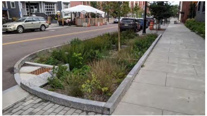
Figure 23. Stormwater retention with rain garden.
