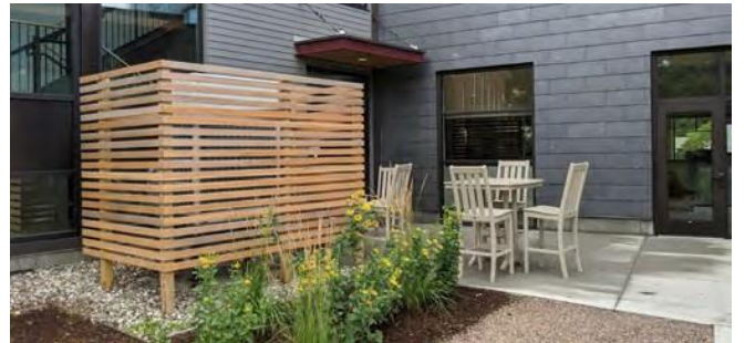
Figure 30. Screening of mechanical equipment.
