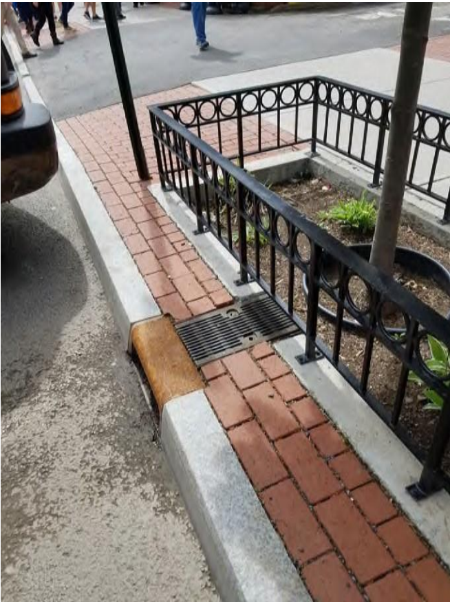
Figure 22. Stormwater retention. This example of stormwater retention captures water from the street and stores it in a planting bed where it waters the plants and trees.
