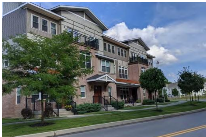
Figure 34. Building massing. This long building is nicely broken up with strong depth fluctuations in the facade and roofline which help to identify individual apartment entrances and create balconies.
