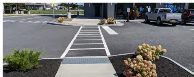
Figure 20. Internal parking lot crosswalk.
