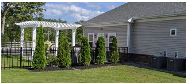
Figure 27. Screening of mechanical equipment.
